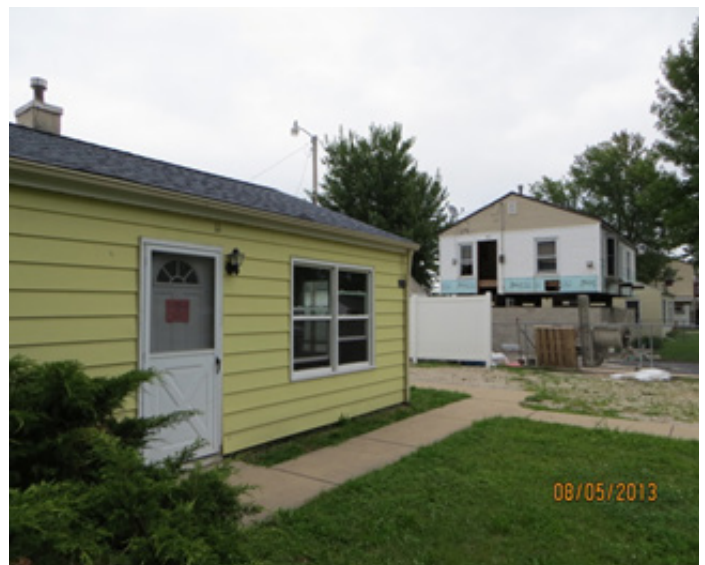
A red-tagged home and a home being elevated in Carbon Cliff after flooding in 2013.
