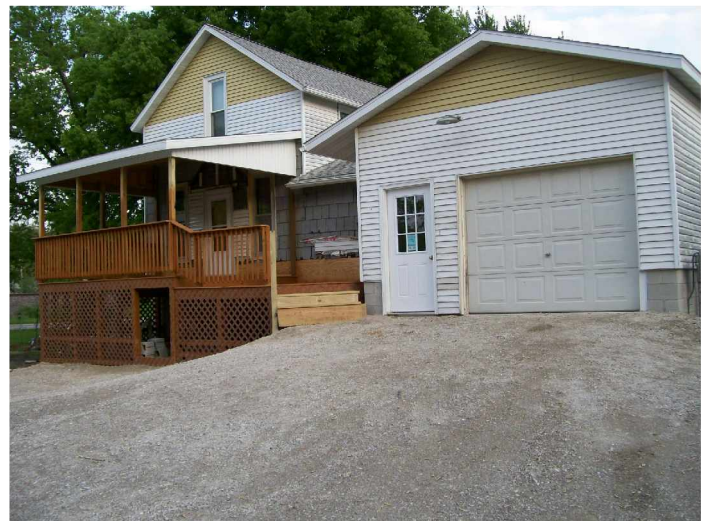
These Before and After photos show a home that was elevated after being damaged by the January flood.
