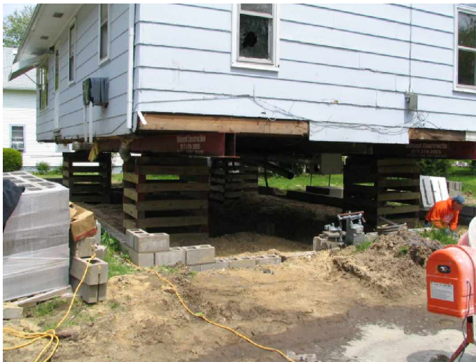
Construction underway to elevate a home in Watseka.
