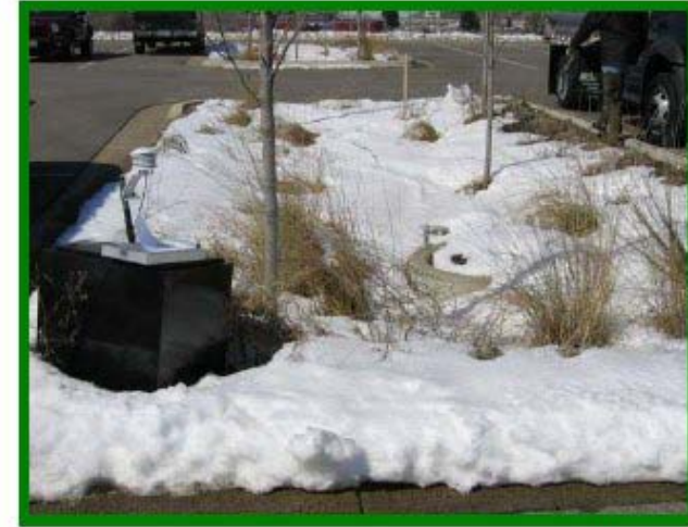
Cottage Grove Bioretention Cell Cottage Grove, MN
