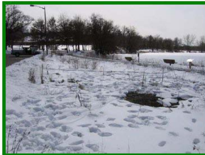
Thompson Lake Bioretention Cell West St. Paul, MN
