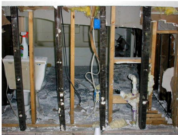
**Figure 16-11: Even standing floodwater can cause substantial damage.**
