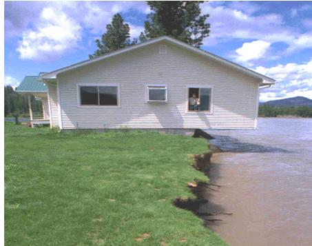
**Figure 1-5: Riverine erosion can undercut structures**
